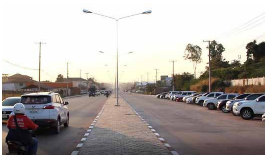
The road linking between the Tanmixay crossroads in Xaythany district and the Sikeuth junction in Naxaithong district, Vientiane, now open for public use following the completion of a major upgrade of this 9.4-km road.
