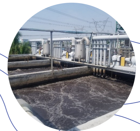
Figure 5.8/ Biological treatment stage of wastewater treatment plant
