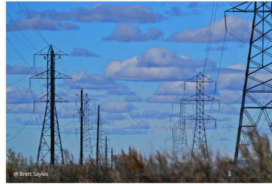
Figure 8.4/ Factory purchases grid electricity for use
